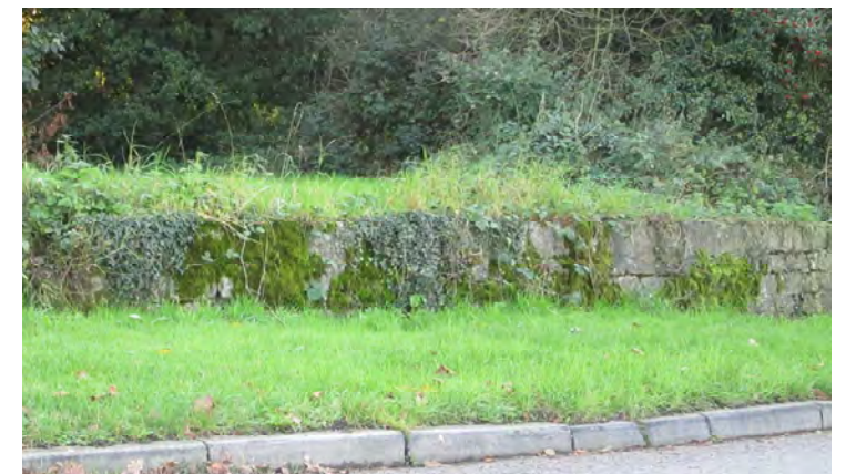
Image of current retaining wall
